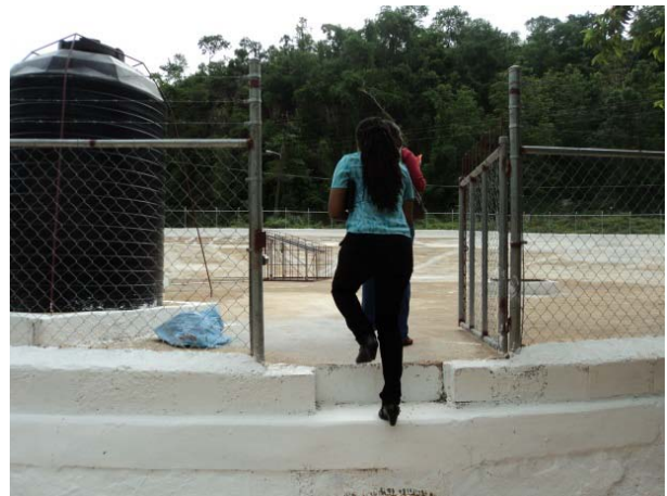
Figure 3: One of the refurbished community communal tanks with a water storage capacity of approximately 100,000 litres (58,000 gallons). Water is used for domestic purposes and is purified in partnership with the Parish Council. Photo by: Hyacinth Douglas, 2013.
