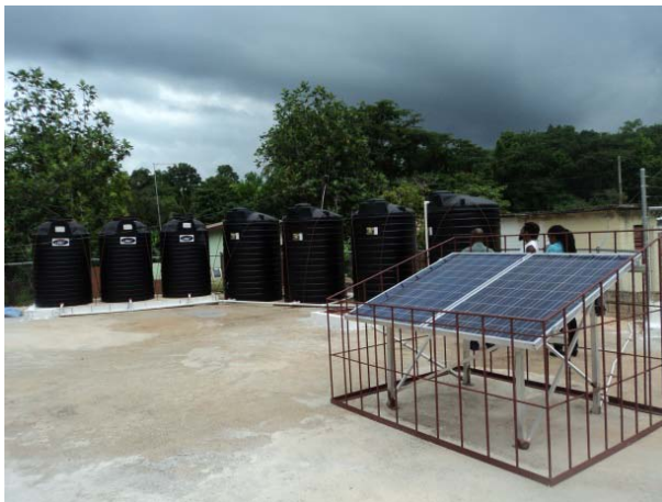
Figure 2: Solar panels are the energy source for the pump. Co-financing provided by the Environmental Foundation of Jamaica. Photo by: Hyacinth Douglas, 2013.
