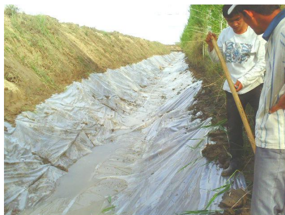
Insulating the channel
