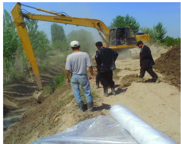
The irrigation channel is levelled to improve water flow
