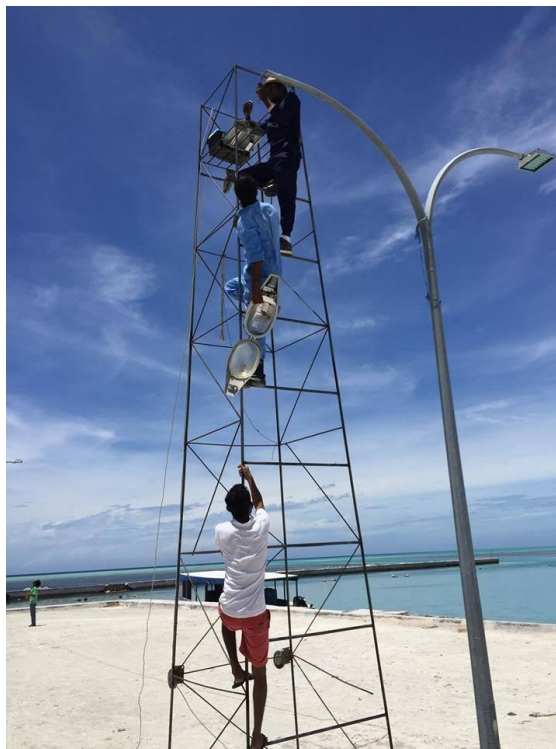
Figure 5: Installation of Energy saving lights
