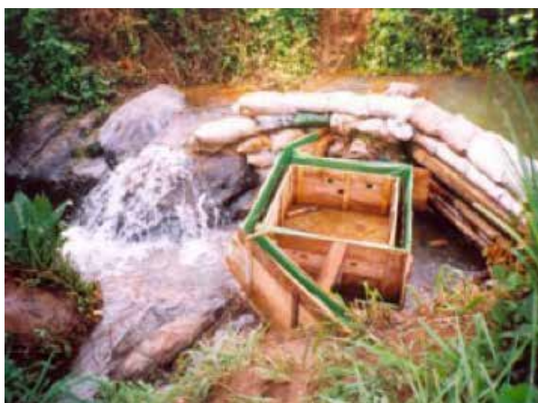
The intake tank constructed by community members
