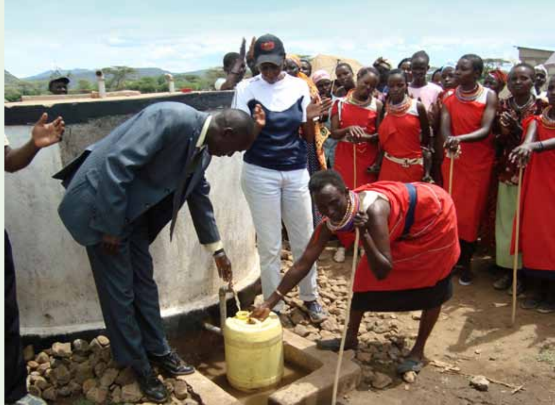
Commissioning of Kailer water project
