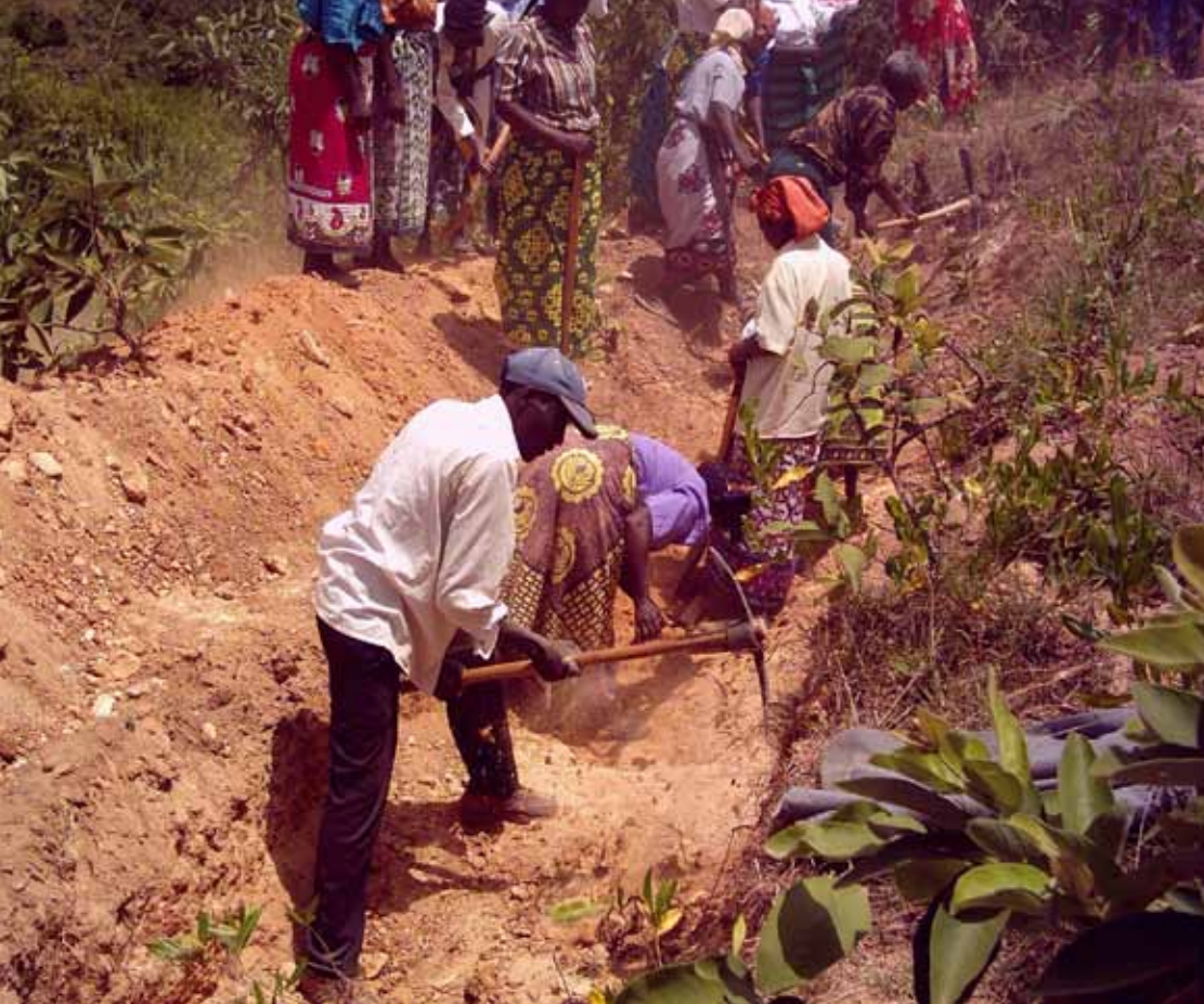
CBO members dig a cut-off trench to reduce soil erosion
