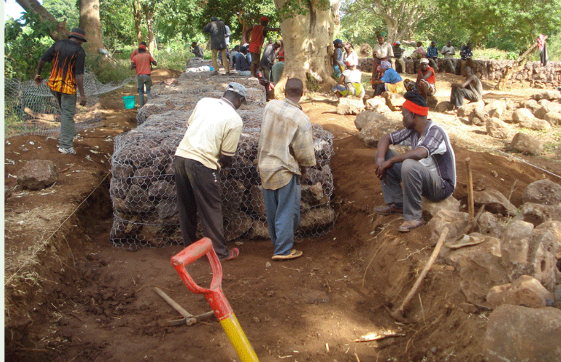
Dyke rehabilitation to protect Njoro springs
