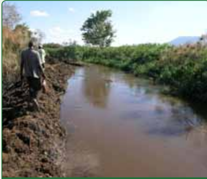
Bank stabilization along River Lumi
