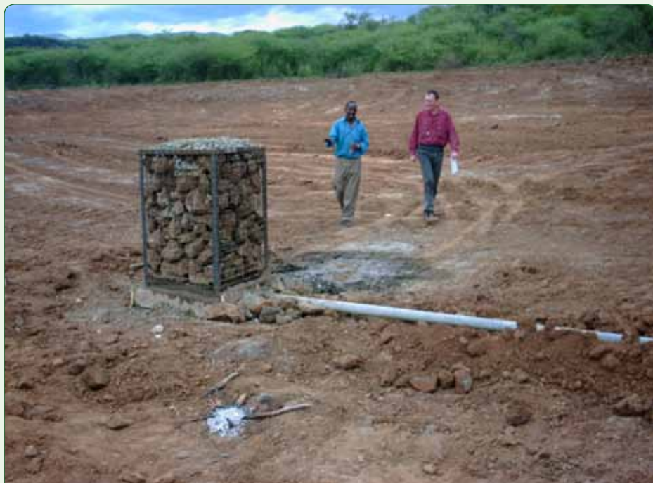
A newly constructed waterpan fitted with a community draw-off pipe
