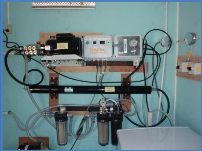
Wind-powered Reverse Osmosis (RO) machine to purify water
