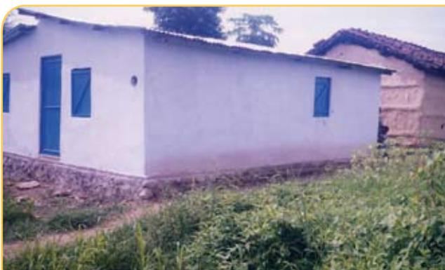
The same completed bamboo house. The house is plastered with cement from both inside and outside the bamboo walls.
