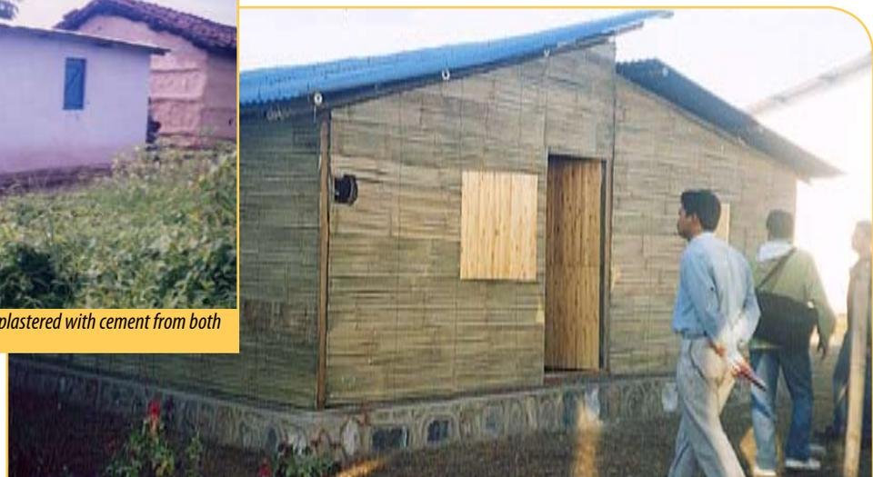
Bamboo house under construction for Kamaiyas in Kanchanpur
