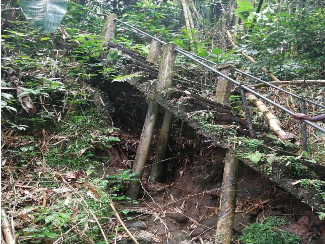
Photo 12 Deteriorating steps leading down to Nanny Falls
