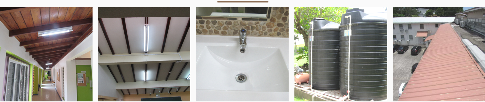
Left to Right: LED lights in the corridors and classrooms; Water efficient taps in restrooms; Water tanks for storage and harvesting; and available roof space for installation of a photovoltaic system. Photos: Barbados Institute of Management and Productivity
