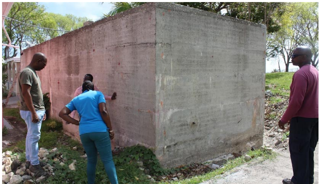
The cistern has the potential to hold 39,000 gallons of water, a more than 5,500 percent increase from the site's current water storage capacity (Photo courtesy Our Lady of Perpetual Help Catholic Church)
