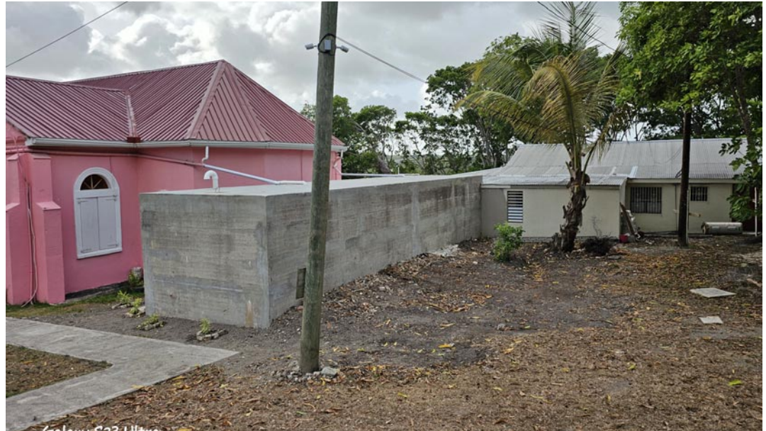
The cistern has the potential to hold 39,000 gallons of water, a more than 5,500 percent increase from the site's current water storage capacity (Photo courtesy Our Lady of Perpetual Help Catholic Church)
