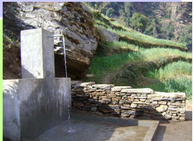
Constructed tap at Tamakot
