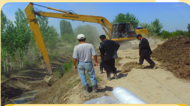
Picture 1. Cleaning of the canal
