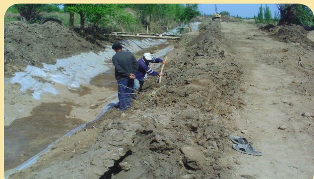
Picture 4. Laying ground
