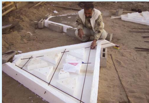
Artificial reef construction — locals poured concrete into models to create triangular pieces (above) which were weighted to the sea floor and later became the perfect habitat for corals (below), photos courtesy of Mr. Sharif Ranjbar.
