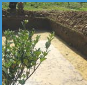
Digging earth for biogas dome
