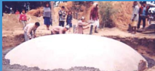
Community biogas dome under construction in Sarlahi
