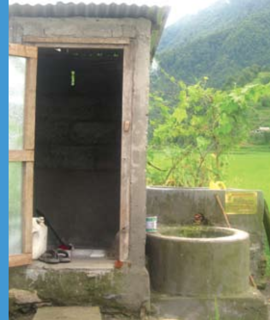
Toilet - attached water hyacinth-fed biogas plant
