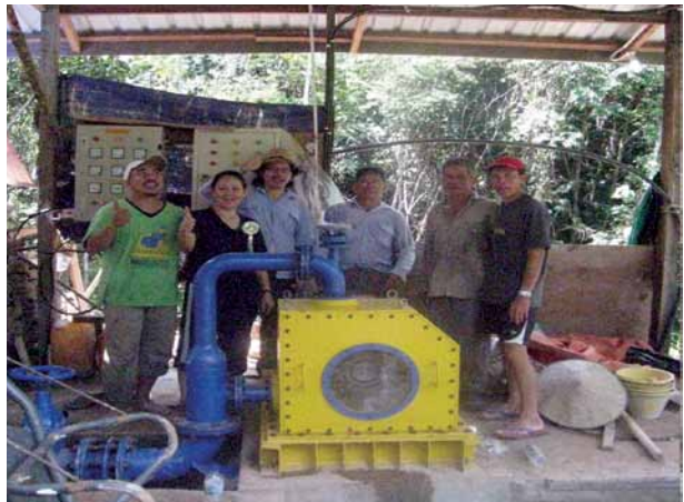
Installation of turbine
