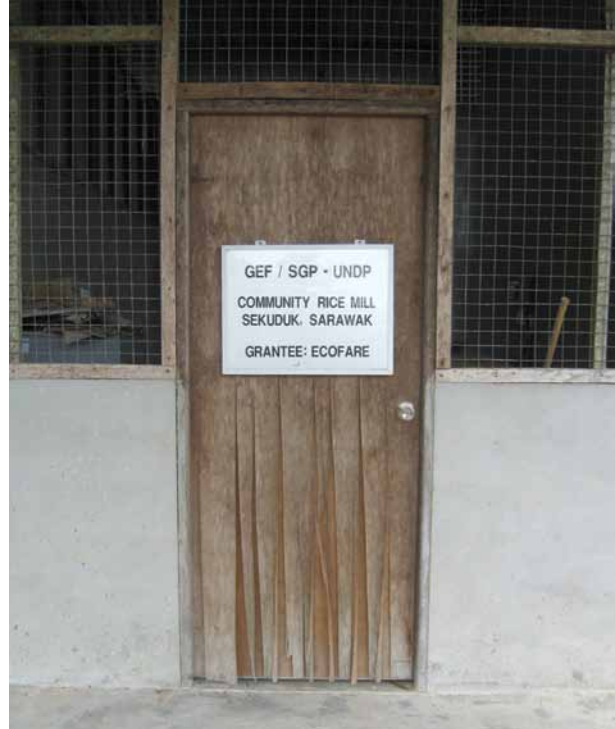
Milling room built in Phase 2
