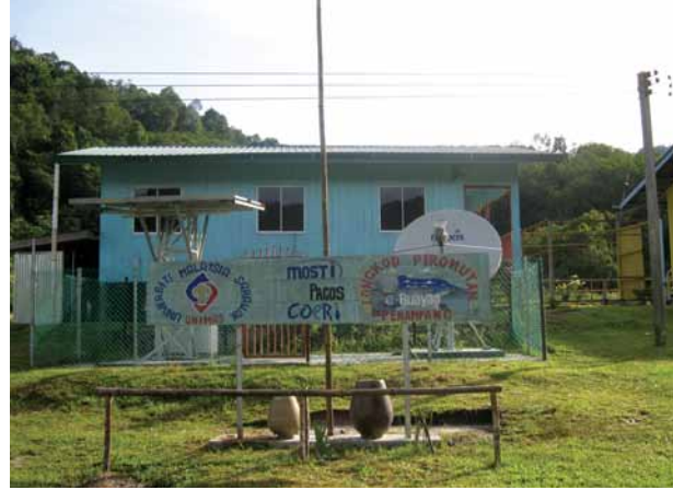
The E-Buayan facility has provided electricity for the whole village.
