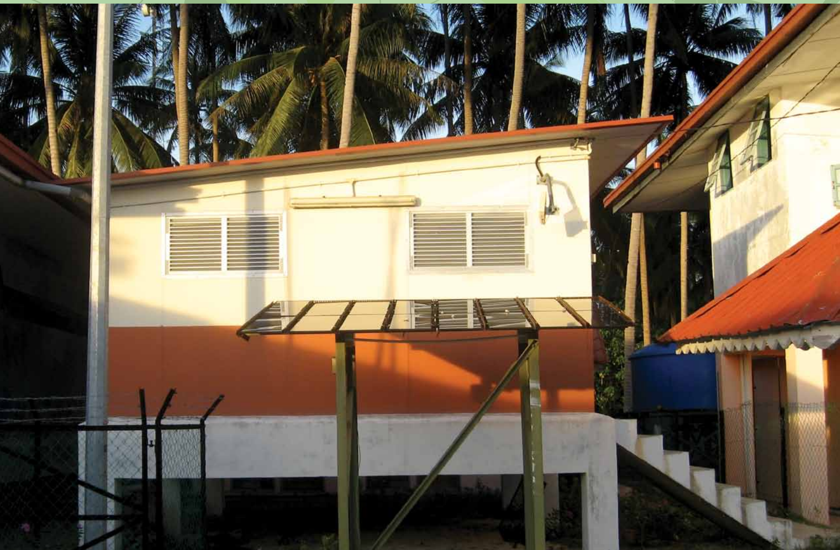
Solar panel installed during project
