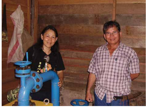
Project staff at turbine room
