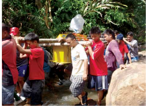
Hauling of turbine and generator
