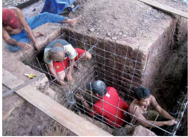
Construction of tailrace and drainage
