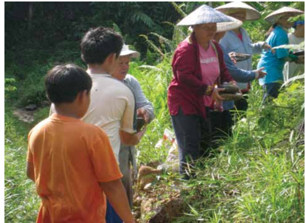
Gathering rocks for reinforcing concrete at micro hydro facility
