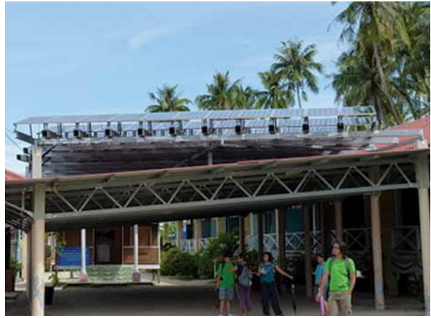
Solar panel (above roof) installed by government
