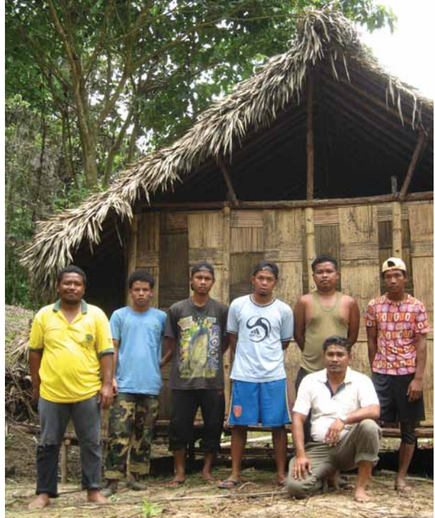
SSN members in front of a ranger's hut under construction
