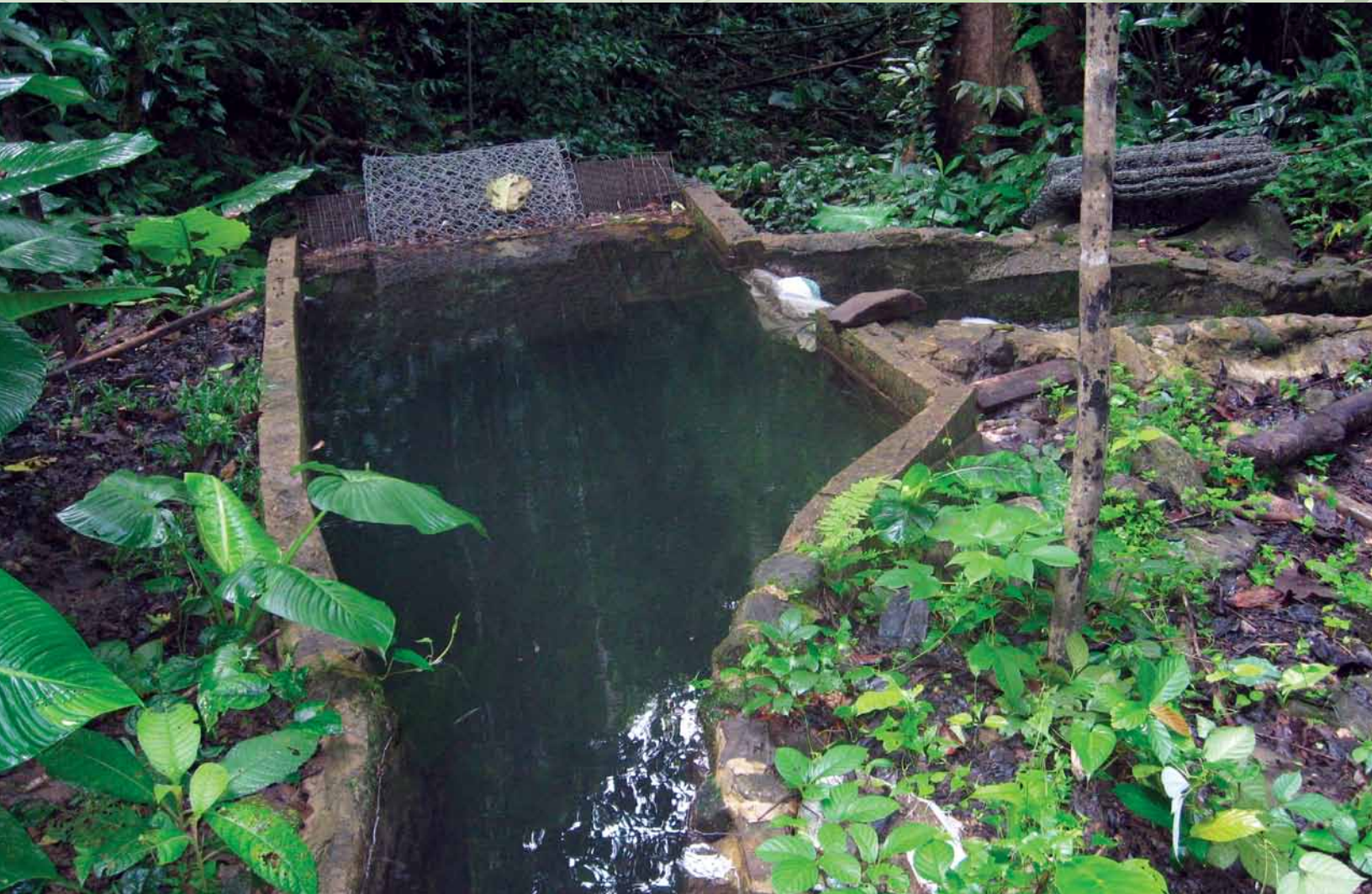
Water reservoir to generate electricity through micro hydro system
