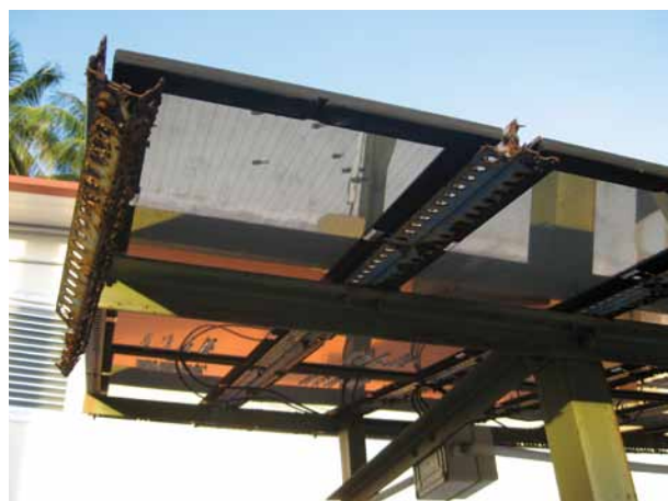
Close-up of solar panel
