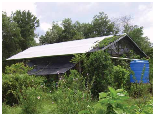
House to facilitate work on demo plot site
