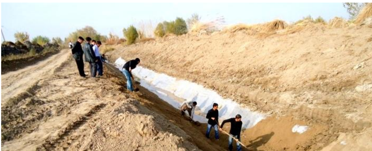
After draining and levelling the channel, community members lined the channel with a PE film to avoid leakage
