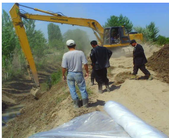
The irrigation channel is levelled to improve water flow
