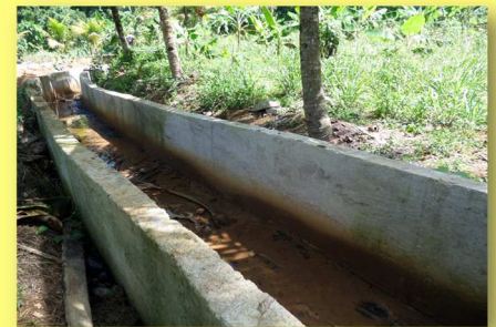
The Storm Drain Constructed in Calibishie
