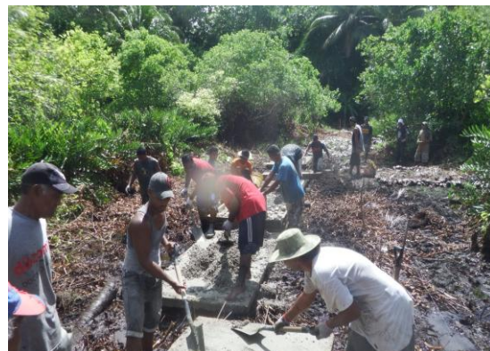
Figure 15: Community members in the Federated States of Micronesia construct blockade structures to protect taro plantations from sea water.
