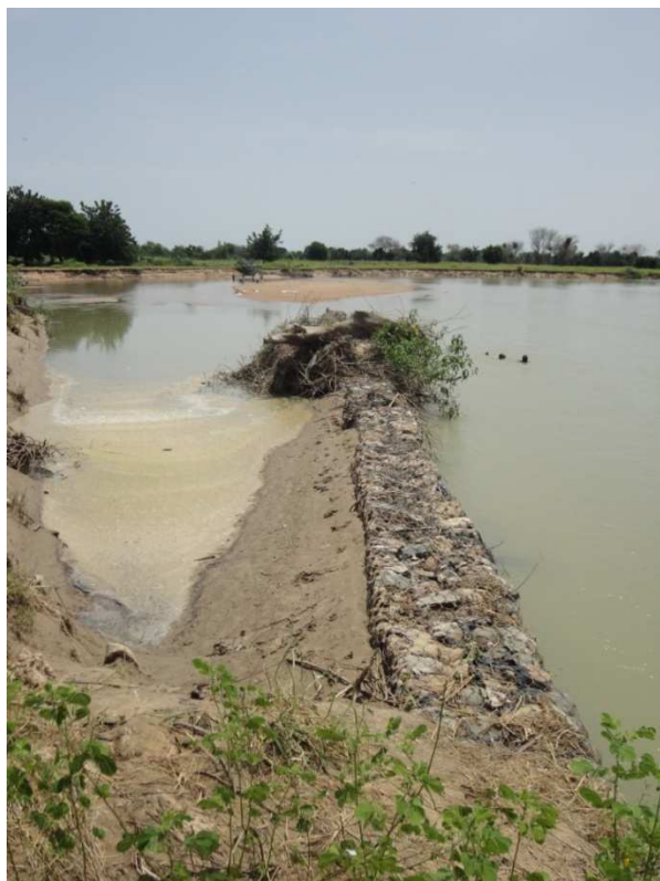
Plate 3b: the threat of erosion within the Mayo Tsanaga course forced the municipal authorities to deflect the bed in order to save the surrounding villages and build a dike to protect the bridge. This dike is now attacked by erosion. Erosion in Balda township at the entry of the lawanat.
