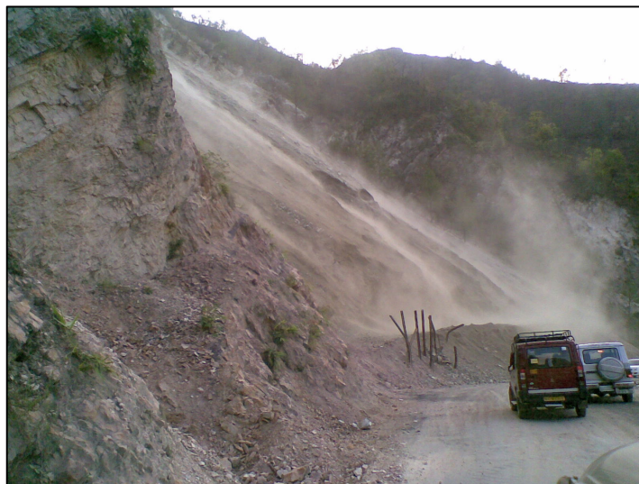
A vulnerable section encountered during travel through Uttarakhand
