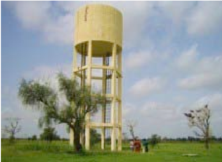
Water storage tower in Bambey, Senegal
