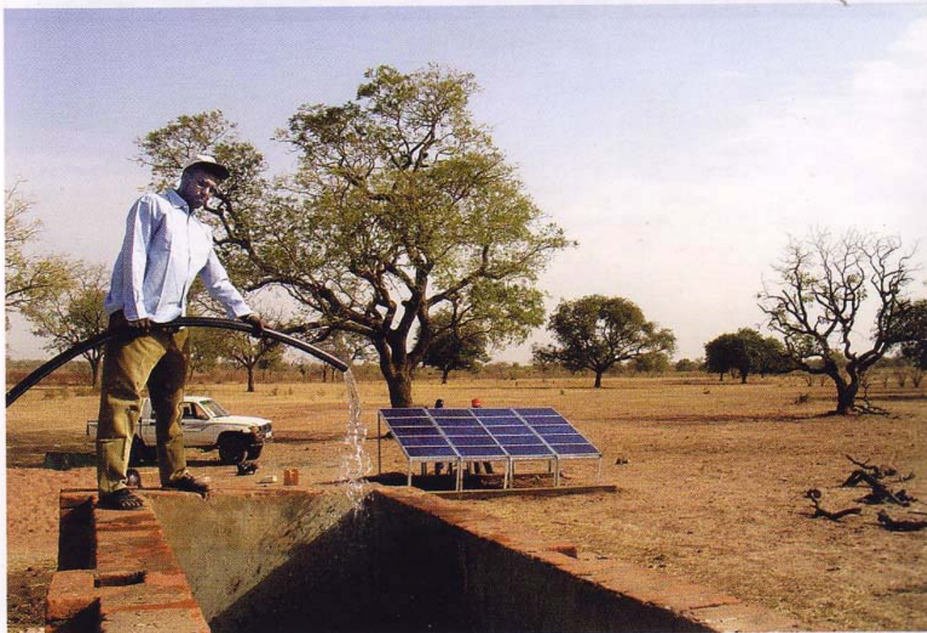
1kW of solar panels complements the wind turbine, with associated benefits of a hybrid system.
